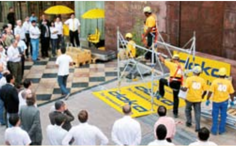
▲ A Doka team assembled a Staxo 40 tower at record speed during the customer event
