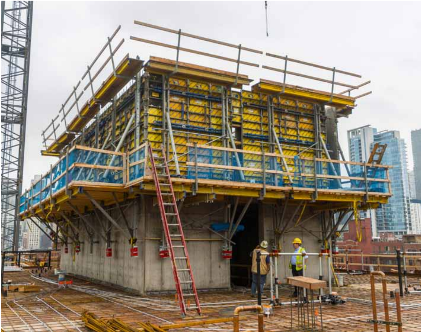
▲ The use of MF-240 climbing formwork is unique in that it was utilized on a job with a small footprint, while in other jobs of this size, alternative self climbing systems are commonly used. However, the contractor wanted to try an alternative, and the MF240 is easily tailored to a wide range of different requirements.
