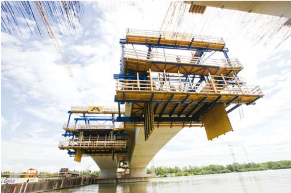
◀ The Cantilever Forming Traveller (CFT) is a completely rentable, all-in-one system offering an optimum construction workflow.
