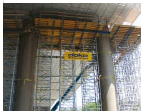
▲ Staxo 100 , a new revolutionary shoring system, is capable of supporting high loads, up to 22.5 kip per leg. Adaptable to any layout, floor shape, and load, the system offers a high level of stability, built-in ladder system, and tie-off points for harness or arrest equipment. The product, winner of the 2010 Most Innovative Product at World of Concrete, is in use on the Alexander Hamilton Bridge in N.Y., supporting pier cap restoration and reaching up to 100 ft. in support height. ◻
