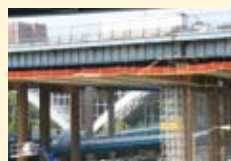
Alexander Hamilton Bridge
