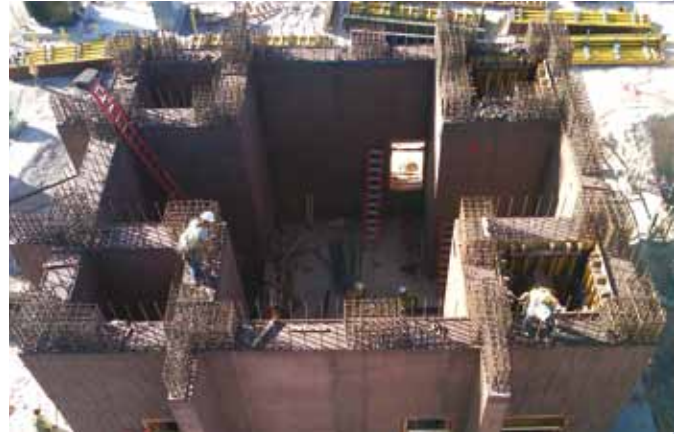
▲ With only three system components, large-area formwork Top 50, is a customizable construction kit where shape, size, tie-hole pattern and form-facing elements can be adapted to suit any requirement.
