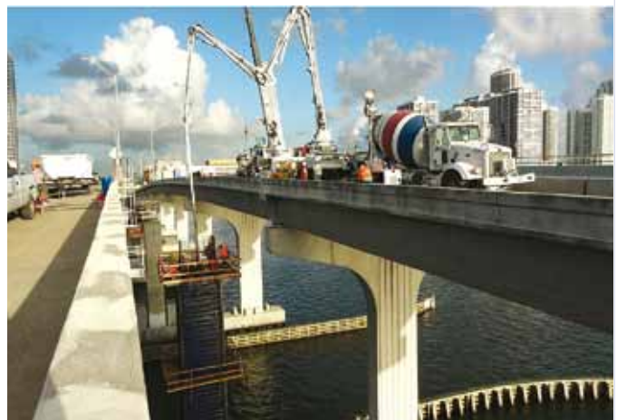
▲ Doka's Steel Girder Form is capable of forming large columns up to 12'-0" x 12'-0" completely tieless.
