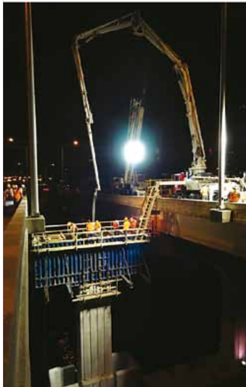
▲ Concrete was poured during night hours when temperatures were cooler to ensure the concrete reached the right strength.
