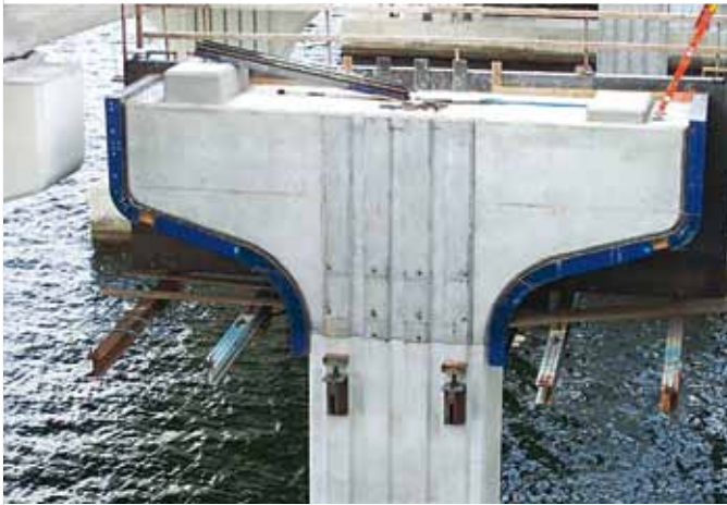
▲ Doka's Steel Girder forms easily stripped in two sections.
