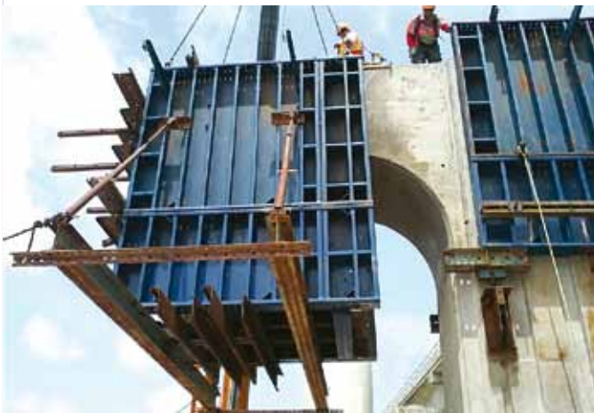
▲ Unlike a typical hammerhead cap, this cap had rustication tying into it from the column requiring a three step stripping process.
