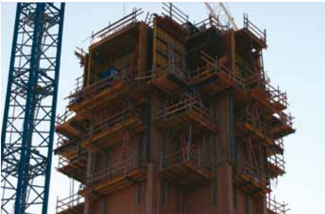
▲ The Top 50 wall system together with self-climbing SKE 50 plus, provides faster completion, maximum safety and a superior architectural concrete finish.
