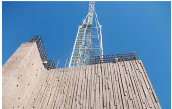
▲ The Top 50 wall system together with self-climbing SKE 50 plus, provides faster completion, maximum safety and a superior architectural concrete finish.
