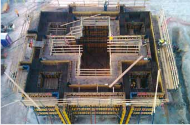
▲ With only three system components, large-area formwork Top 50, is a customizable construction kit where shape, size, tie-hole pattern and form-facing elements can be adapted to suit any requirement.
