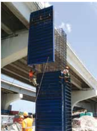
▲ The three main parts of the columns on the water included the stub wall, column, and pier cap, all formed using steel girder formwork.
