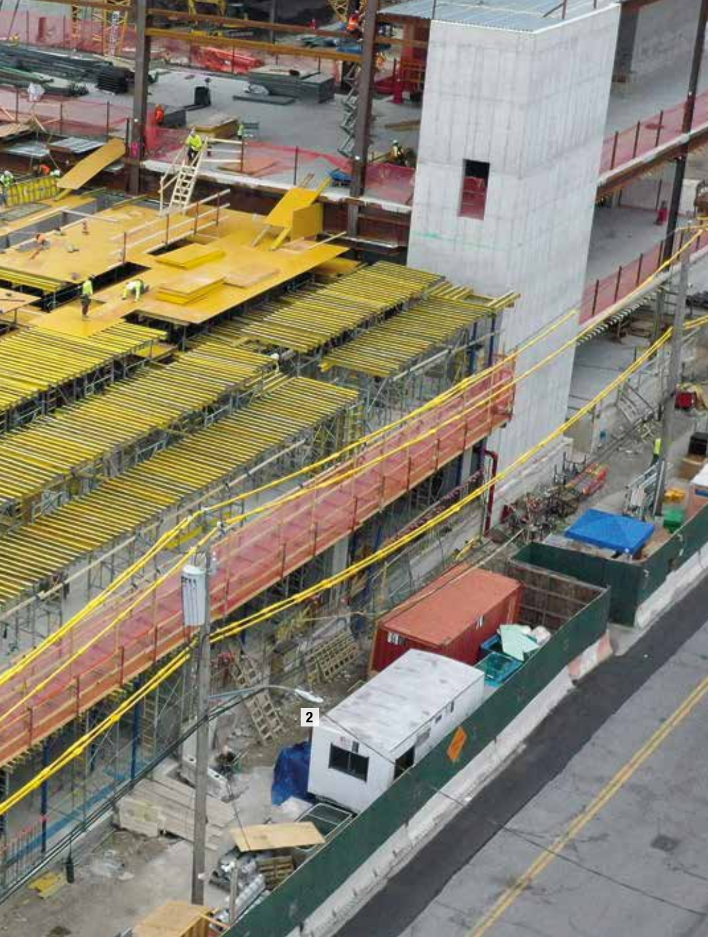
Approx. 52,500 sq. ft. of Doka shoring installed
