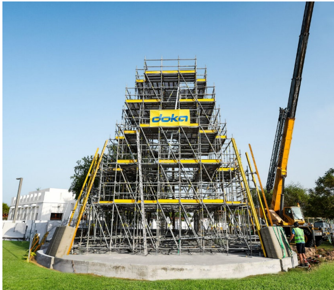
Doka's Ringlock system cocoons the "Smart Qatar" Pavilion.
