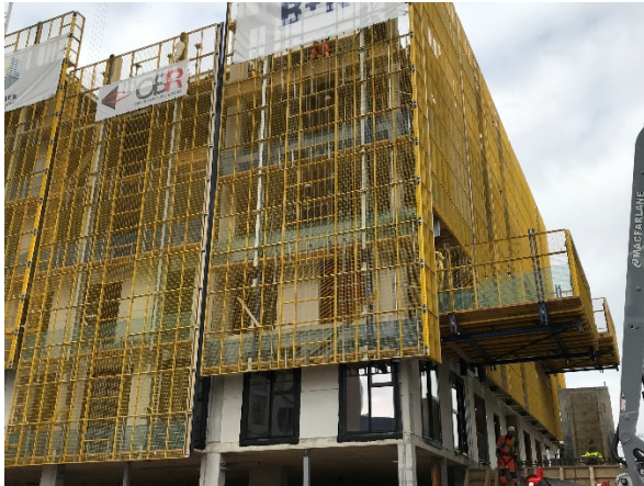
Waterproofing and Window units installed following the first movement of the screens
