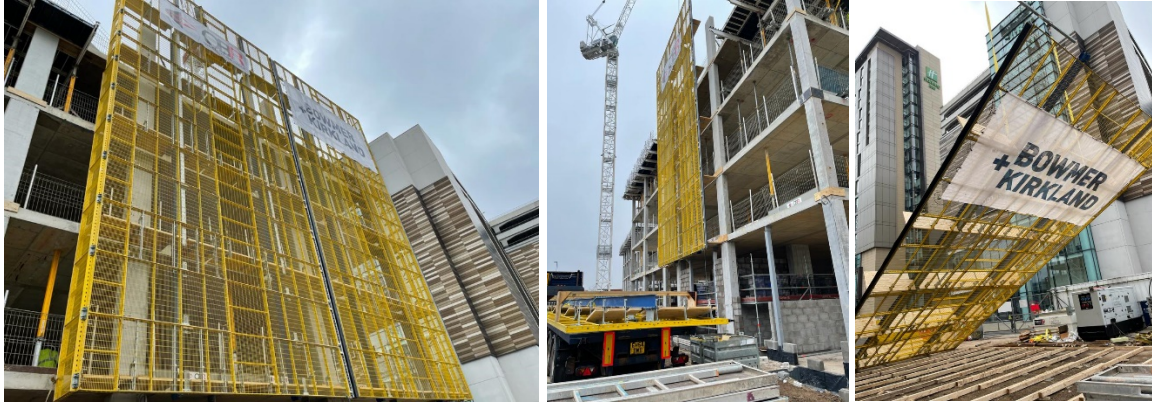
Installation of the Xclimb Protection Screens in progress from the first floor
