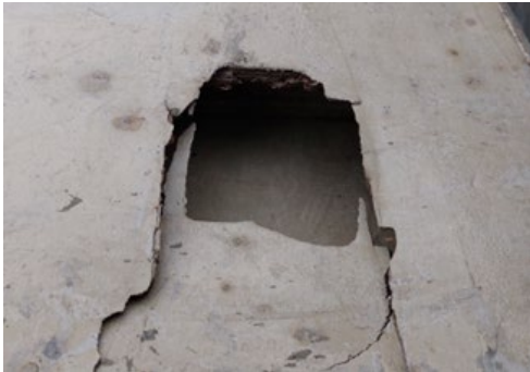
Holes + drills diameter > 2 cm
