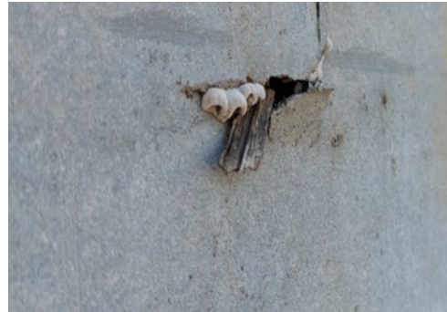
Holes + drills diameter > 2 cm
