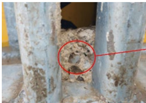
Anchoring impossible
