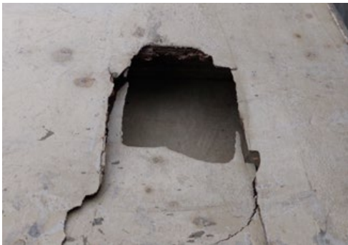
Gaten + boringen diameter > 2 cm
