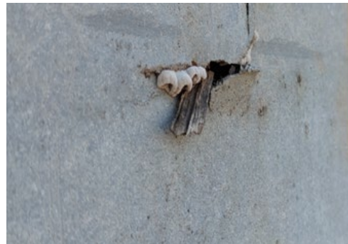
Gaten + boringen diameter > 2 cm
