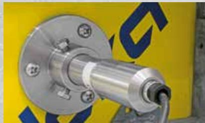
The wall sensing element for the cable sensor is incorporated directly into the form-facing and repositioned together with the formwork.
