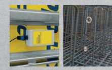
The cable sensor has up to three measuring probes and is positioned on the reinforcement before the concrete is poured.
