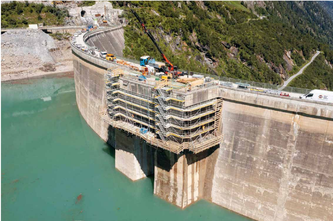
That’s a hit: Doka’s formwork and scaffolding operate seamlessly under high alpine conditions.
