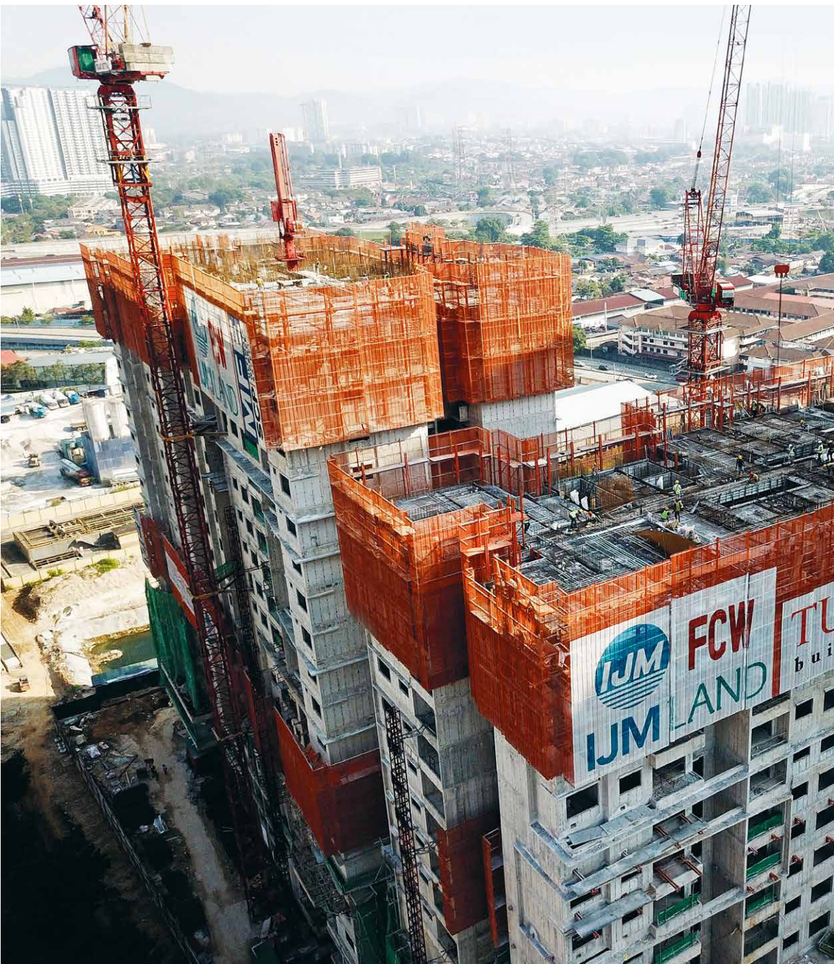
Protected at height: The Self-Climbing Platform with integrated protection screens progresses floor by floor with the structure.
