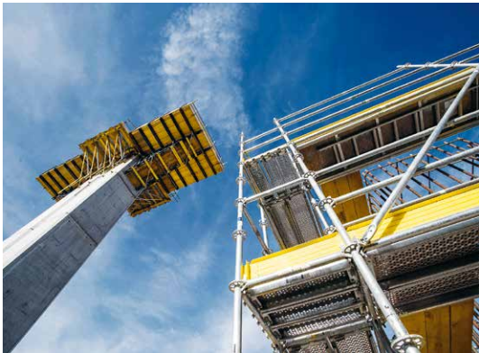
Formwork and scaffolding from a single source for the Zdíky Viaduct in Czechia.
