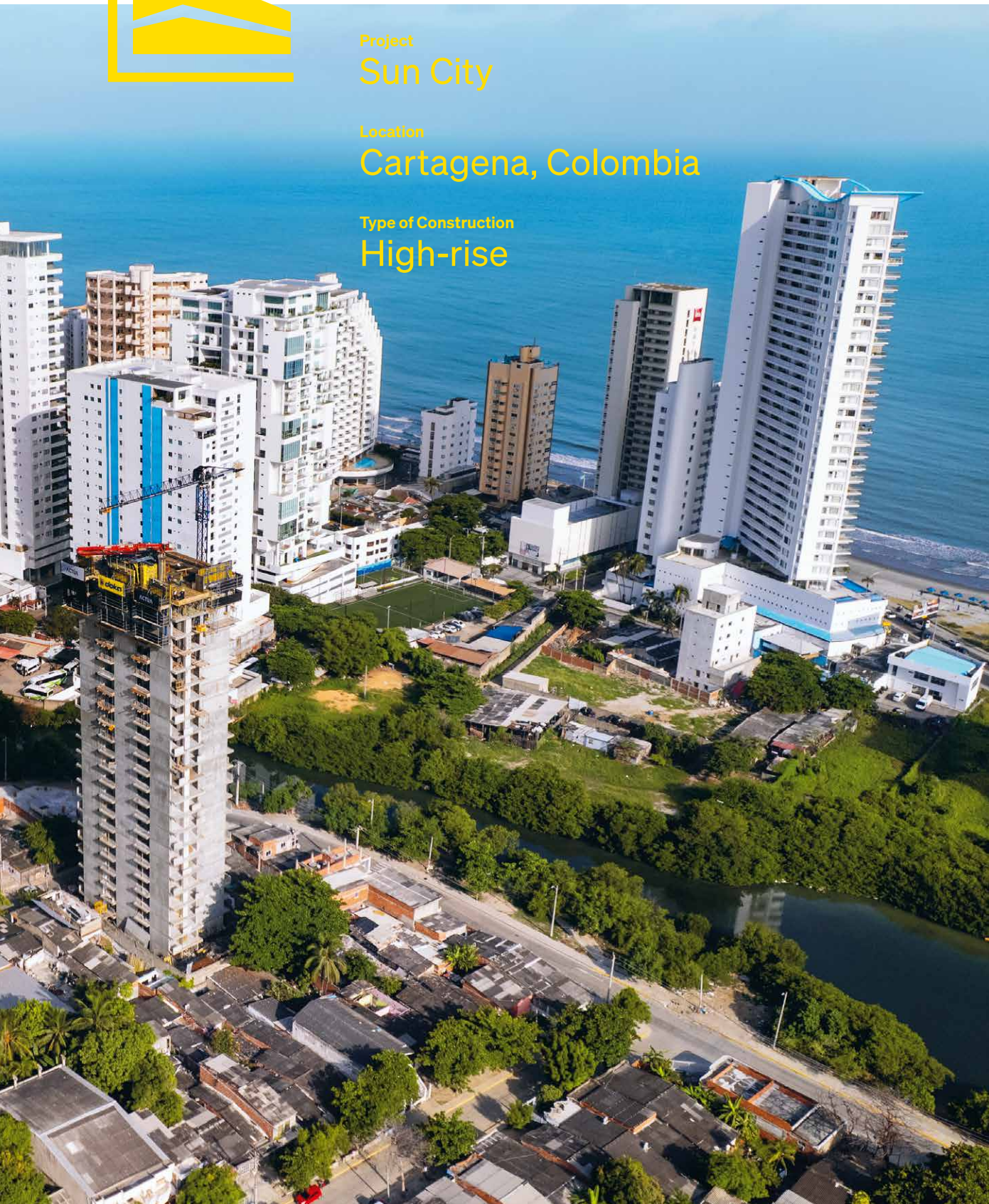
Sun City: Smart climbing solutions enable efficient high-rise construction in tight spaces.
