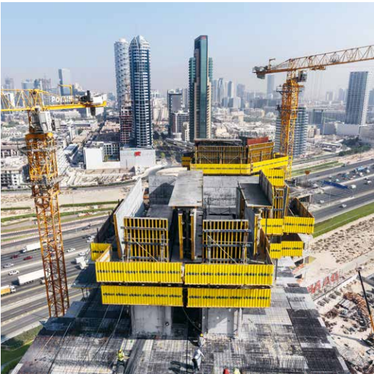
Automated climbing formwork SKE50 plus enabled crane-independent and steady vertical core-wall construction.
