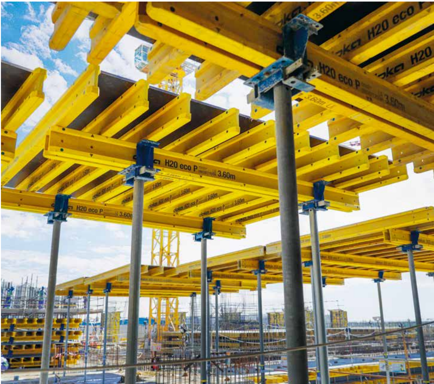
Doka's workhorse timber formwork beam H20 eco P was used extensively throughout the project.
