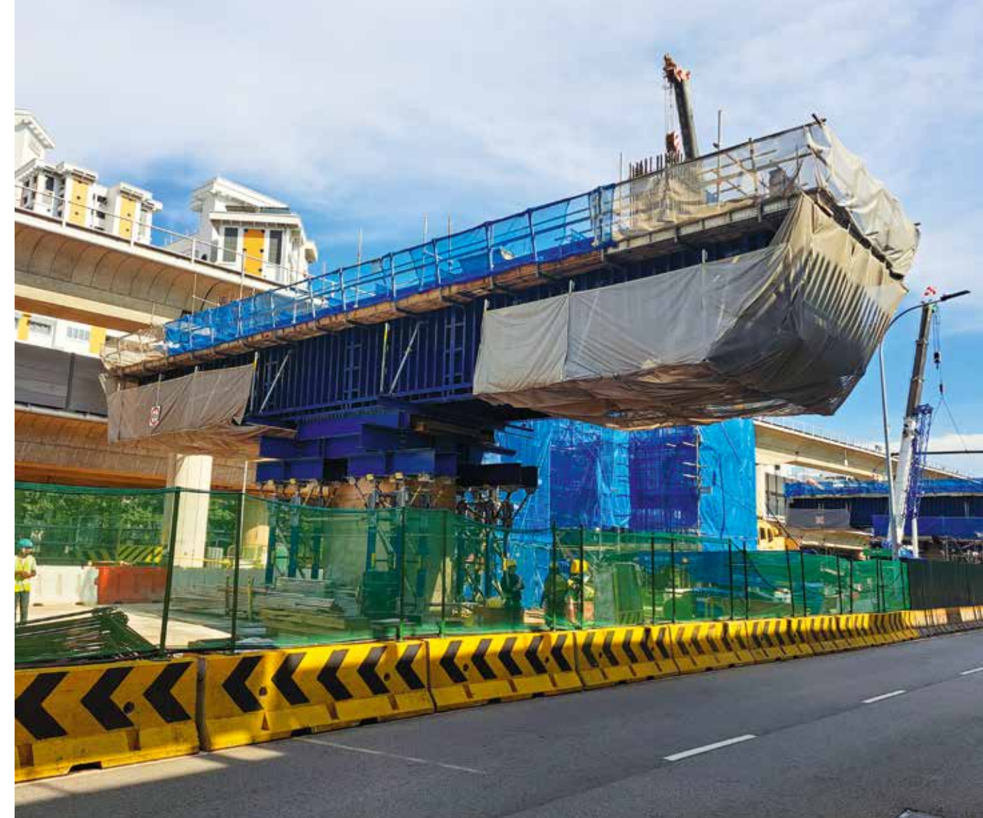
Following just one night of road closures, Doka's Steel Girder Formwork and UniKit shoring tower ensured a key stage of the Toh Guan Station was completed on time and on budget.
