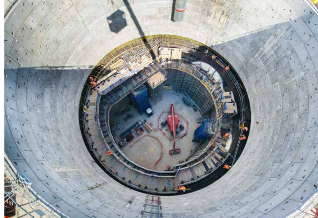
View from the top of the HS2 shaft at Victoria Road onto the Doka-formwork
