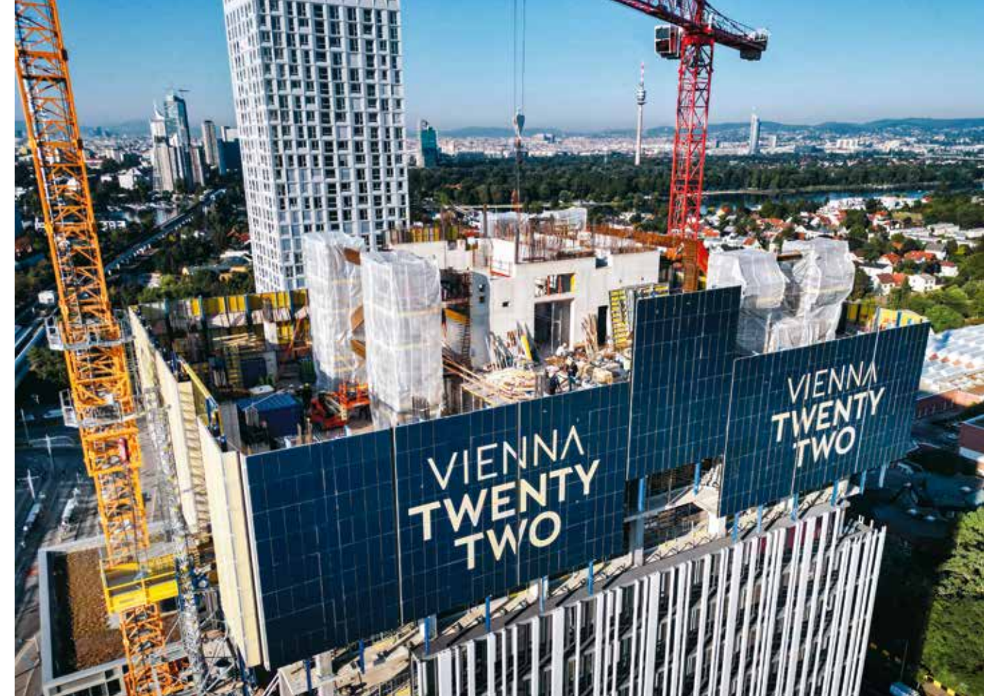
With its Protection screen Xclimb 60 and Ringlock modular scaffolding, Doka met the highest demands in terms of construction progress, safety and precision.
