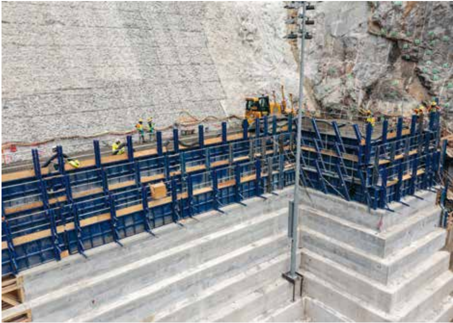
New dam steps are formed using Doka’s custom girder system.
