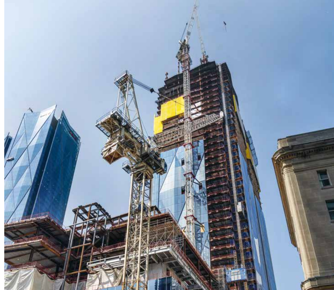
Making its debut in Canada, the Doka Xbright screen enhances safety while adding a splash of yellow to Toronto's skyline.
