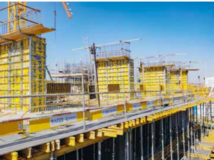
Framed Formwork Frami Xlife, ideal for fast and economical forming, was used for columns, core and shear walls.
