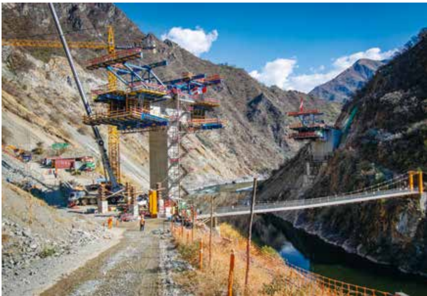
Safe and efficient construction: With Doka's Cantilever Forming Traveller, steady progress was ensured.
