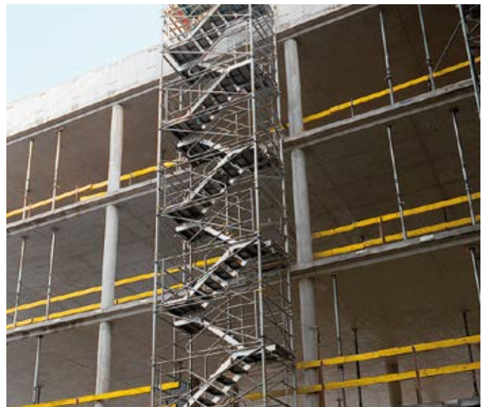
Lightweight, pre-assembled aluminum stair units with non-slip grooved treads for safe and fast assembly.
