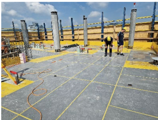
DokaXdek elements were used in the Quadrill project in Austria to easily create the numerous critical fitting areas due to the complex geometric shapes of the building shell.
