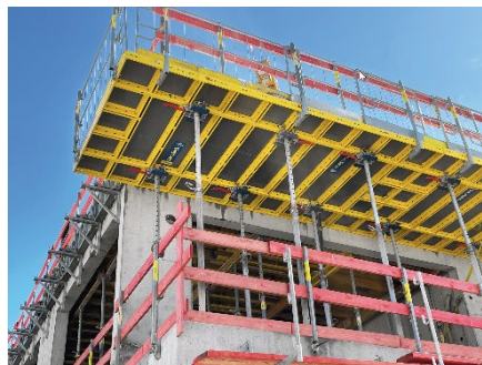
On the Heidepark project in Munich, the DokaXdek tables were also used to support the precast balcony elements.
