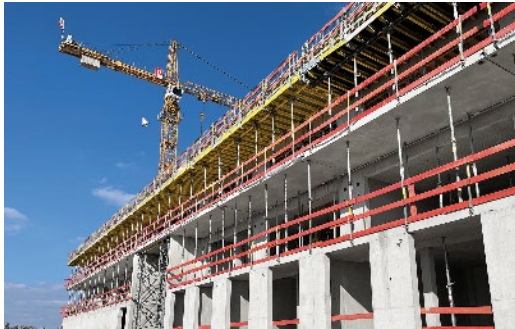
On the Heidepark project in Munich, the DokaXdek tables were also used to support the precast balcony elements.
