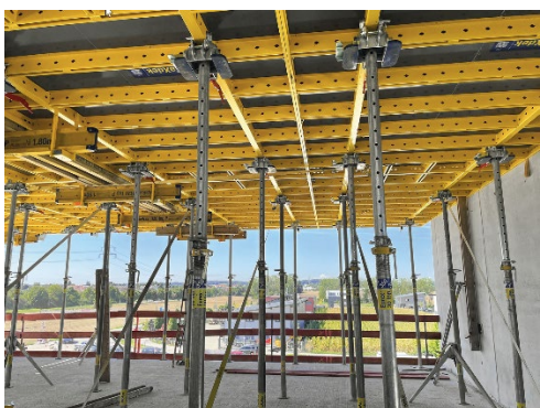
DokaXdek tables were used in the construction of a new four-storey commercial building in Augsburg, Germany.
