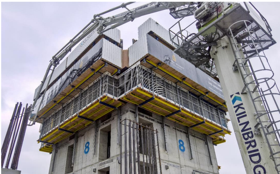
Wood Wharf A3 taking height in preparation for the tenth wall pour with Doka's SKE 50 Plus
