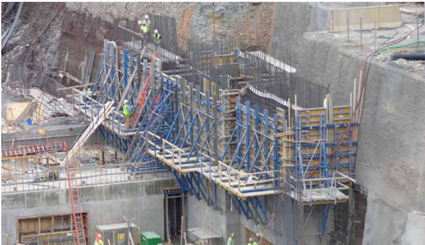
▲ Dam Formwork D22 and Framax are the perfect combination for these tieless one sided walls.
