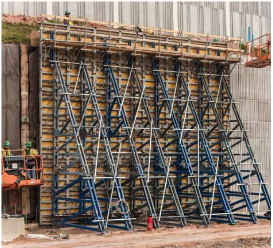
▲ The Framax panels were re-used from structure to structure which made forming super cost-effective.
