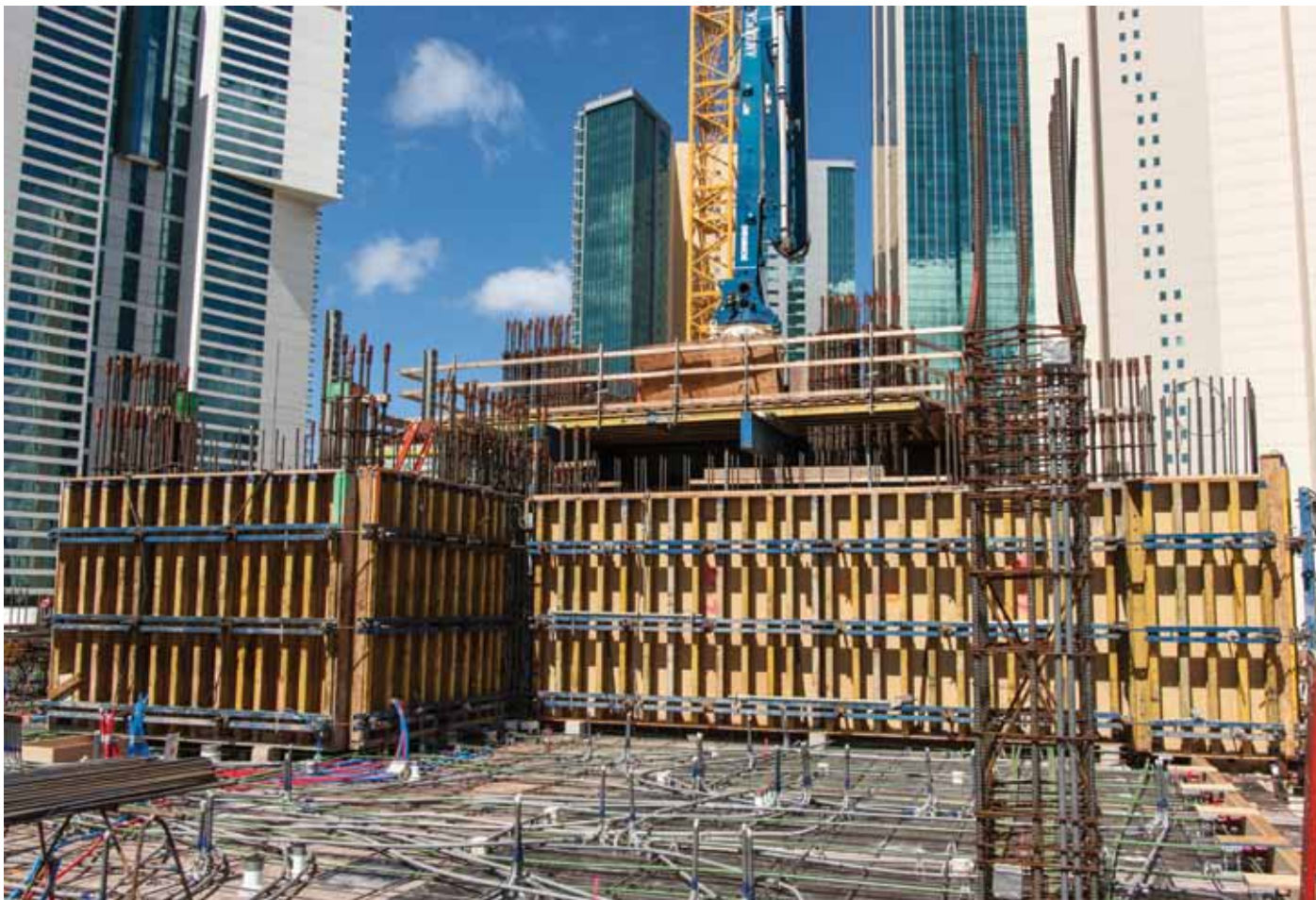
▲ Top50 wall formwork is built to meet the specific dimensions and concrete finish requirements of the structure.
