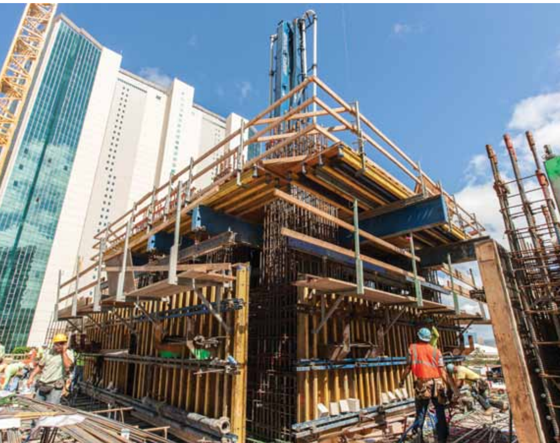
▲ All formwork and placing boom rise at the push of a button with Doka Super Climber.
