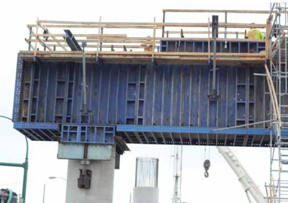
▲ The modular Doka Steel Girder Forms can be ganged and picked in very large sections.
