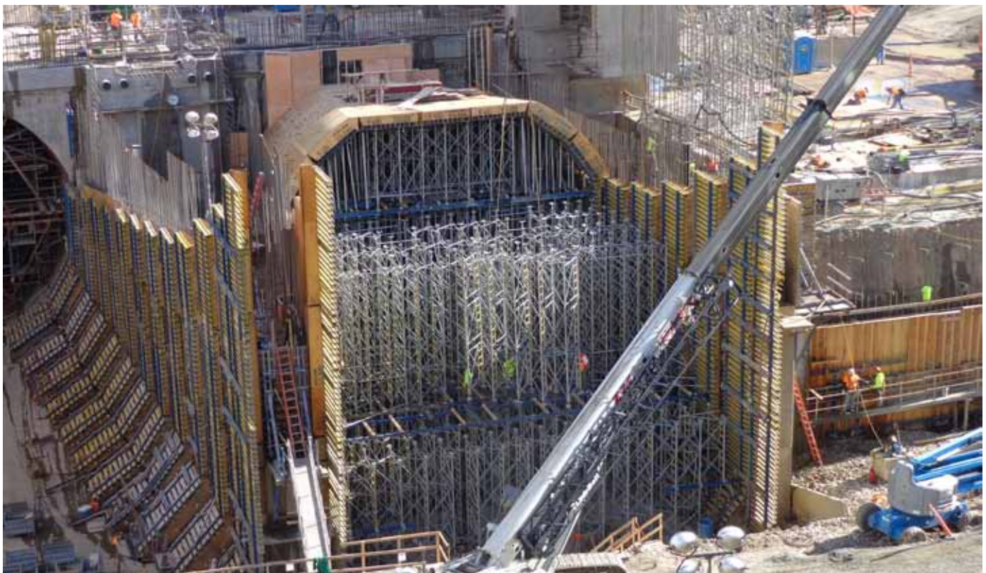
▲ The high load capacity of Staxo100 provided support for the heavy concrete loads and reduced overall material requirements.
