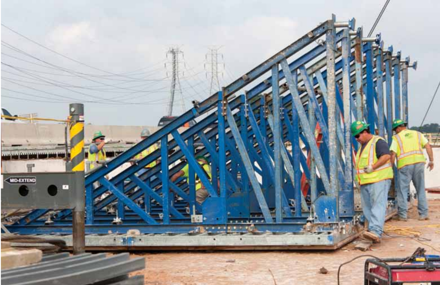
▲ Modular Framax and Supporting Construction Frames are easily assembled into large units at the jobsite.
