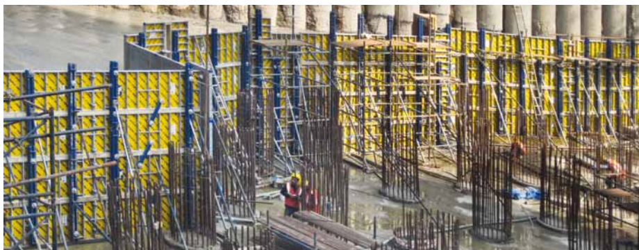
Project: Nathani Heights Location: Mumbai Contractor: Gammon India Pvt. Ltd Structure: Retaining wall
