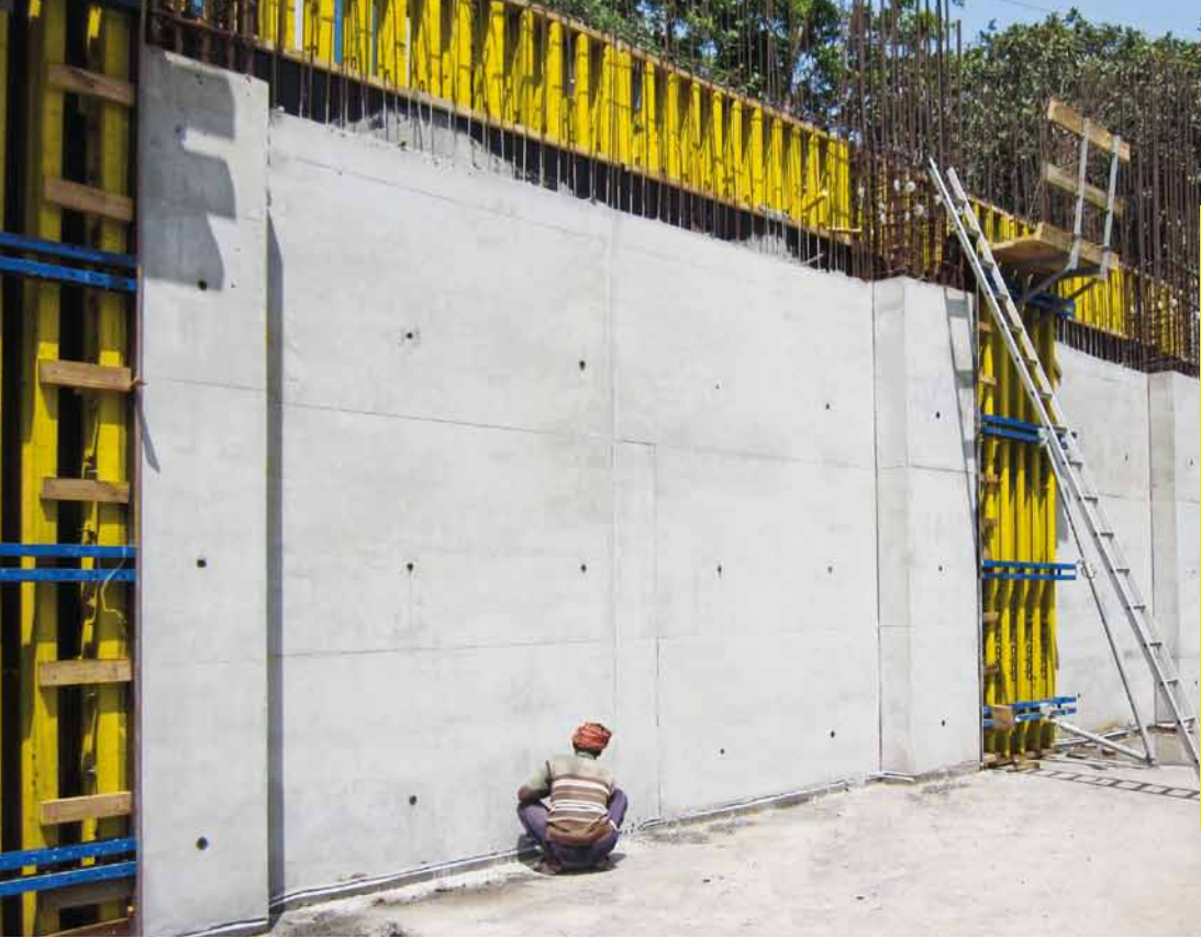
▲ Wall formwork Top 50 was designed to perfection in order to obtain the concrete pattern designs set by the architecture
