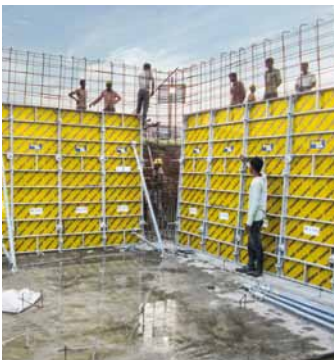
Project: Bannari Amman sugar Mill Location: Karnataka Contractor: URC Construction (P) Ltd Structure: Retaining Wall
