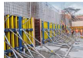
▲ Large area formwork Top 50 being used for retaining wall casting
