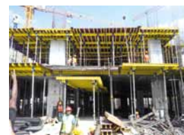
▲ Dokaflex tables being erected at the site
