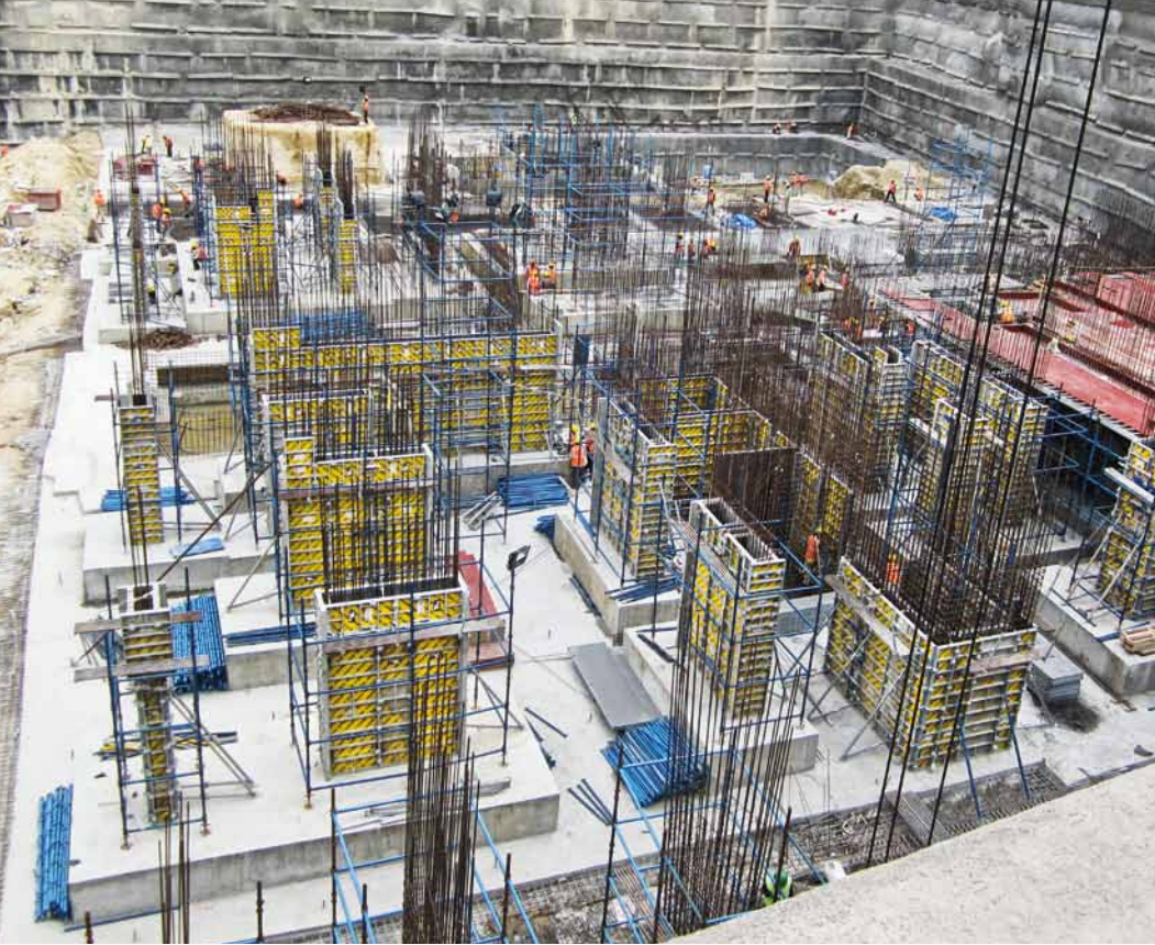
Project: Godrej platinum Location: Bangalore Contractor: Gammon India Limited Structure: Shear walls, column
