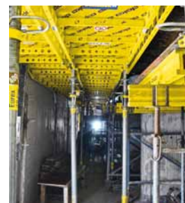
▲ Panel slab formwork Dokadek 30 is handled slab formwork system.
