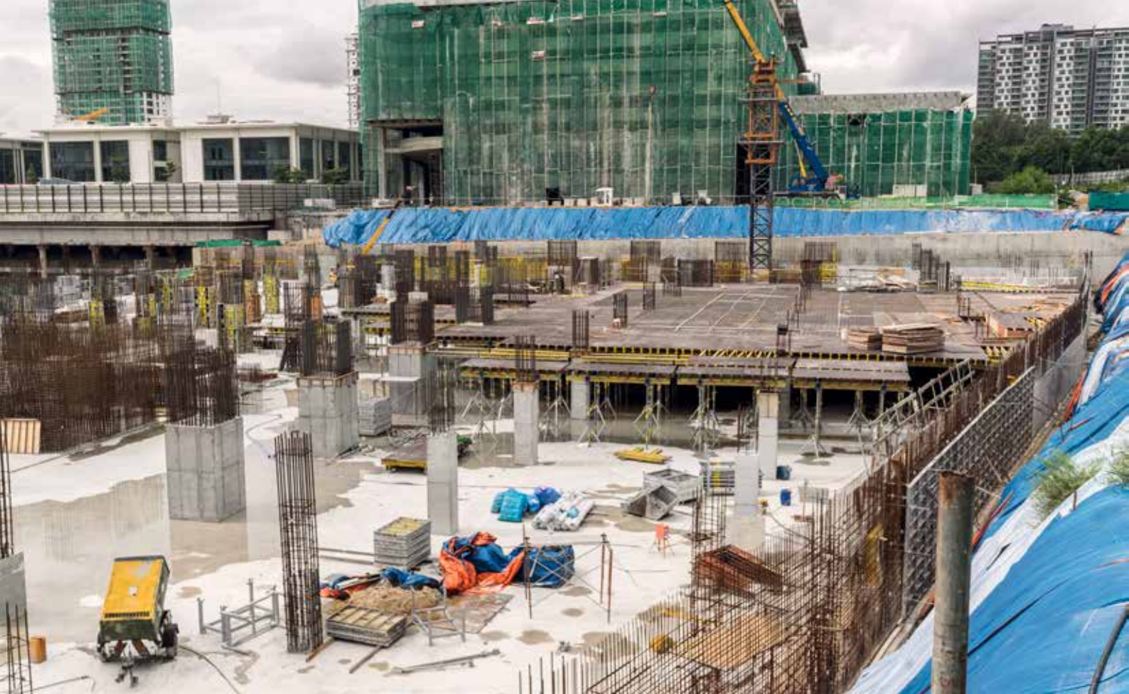
▲ Doka supplied total formwork solutions for slab, column, wall and corewall
